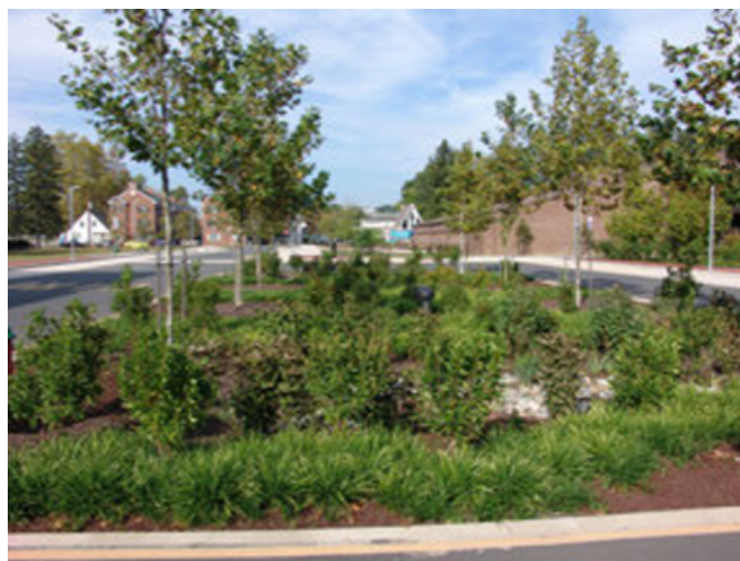
Recently installed rain garden at the University of Delaware's Louise and David Roselle Center for the Arts.
