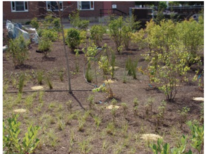
Cores drilled through a hard pan and filled with gravel allowed the area to drain more rapidly. Masses of perennials thrive in the lowest areas.
